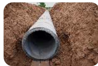
SEWAGE PIPE LINE
